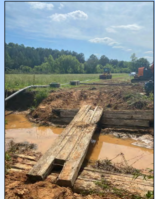
Repairing gravity sewer
