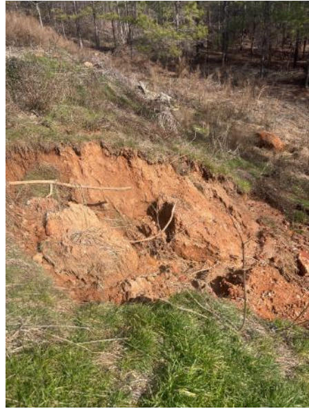
Photopoint 01: 34.68647, -83.15656 Small landslide just downhill of parking lot.
