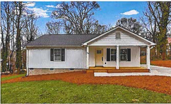
118 Leathers Street New Construction Completed in 2023
