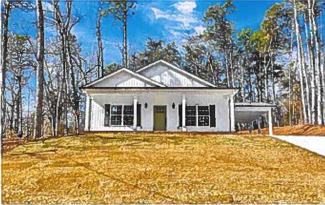
450 Lucky Street New Construction Completed in 2024
