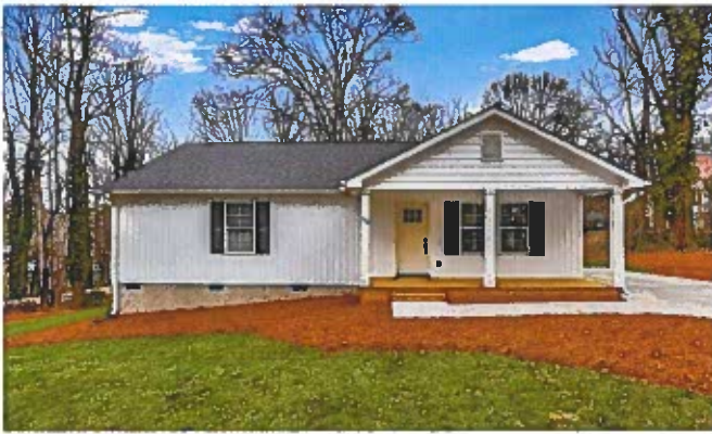
118 Leathers Street New Construction Completed in 2023
