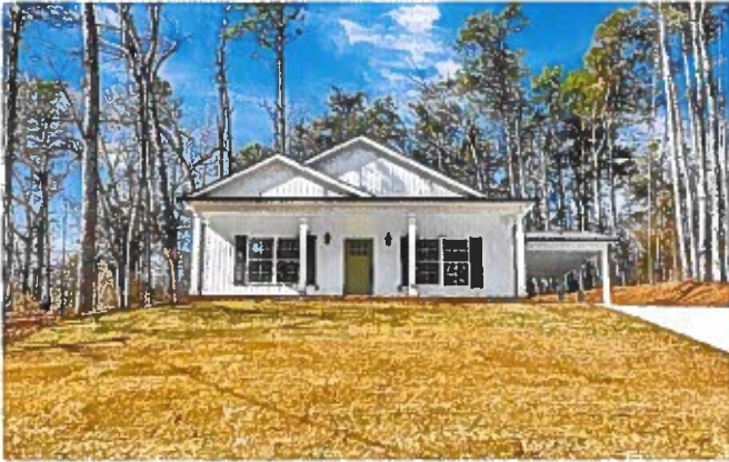
450 Lucky Street New Construction Completed in 2024
