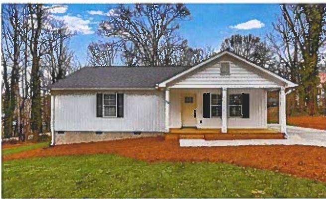
118 Leathers Street New Construction Completed in 2023
