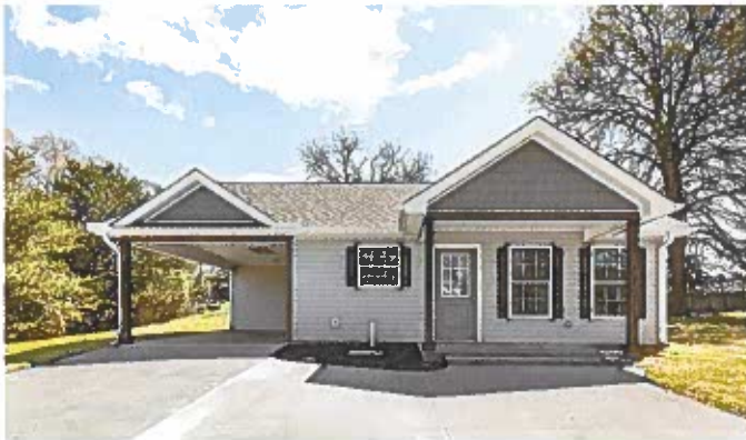
209 Dickson Street New Construction assisted with in 2020
