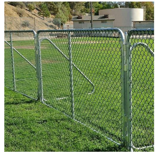
4' Temporary Fence (chainlink)
