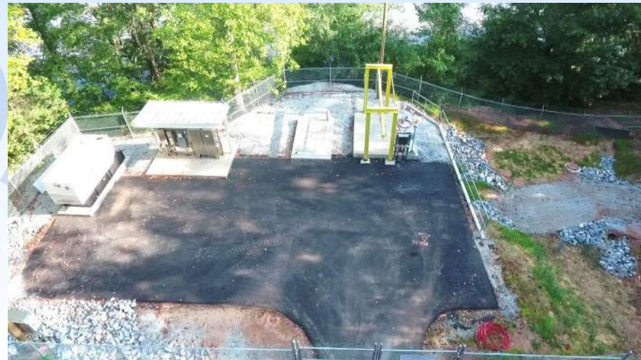
New Duck Pond Pump Station (replacement of Flat Rock PS)
