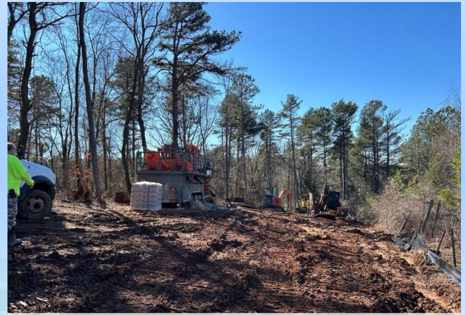
I-85 Sewer Phase II: Installing force main in right-of-way
