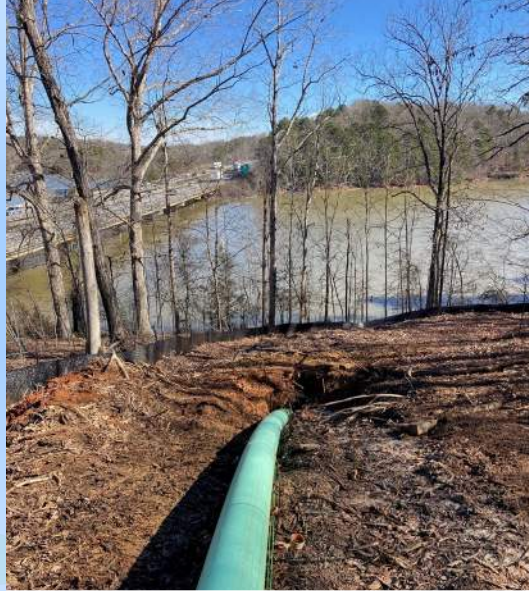
I-85 Sewer Phase II: Pulling force main pipe beneath lake
