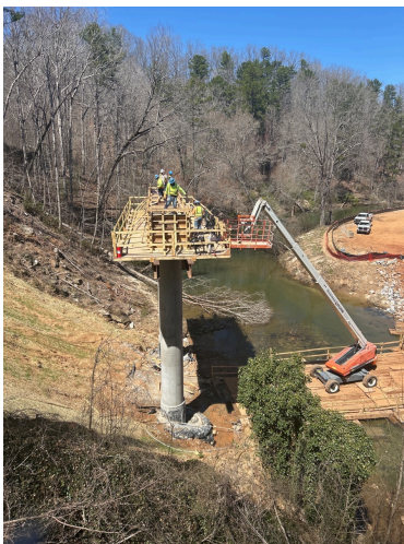
Photopoint 03: 34.68535, -83.15196 Crane and bridge construction in progress.
