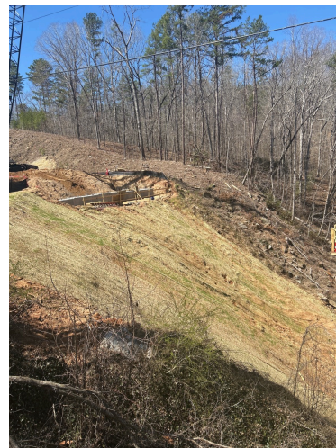
Photopoint 03: 34.68535, -83.15196 Erosion control blanket along disturbed slope.
