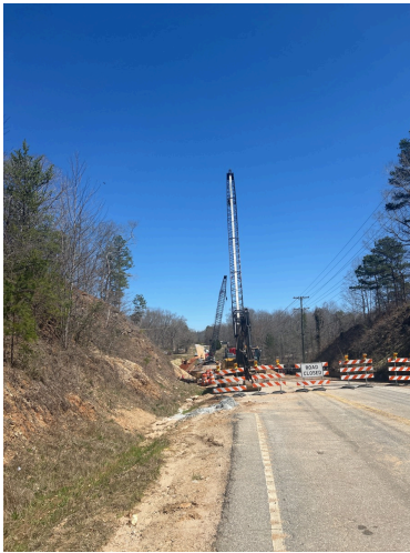
Photopoint 02: 34.68514, -83.15296 View towards Highway 76 bridge.
