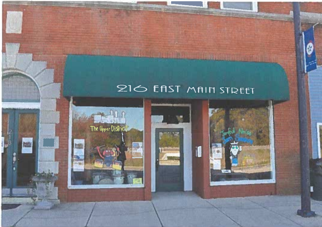
Front Elevation of 216 East Main Street.
