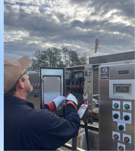
Staff performing work on control equipment
