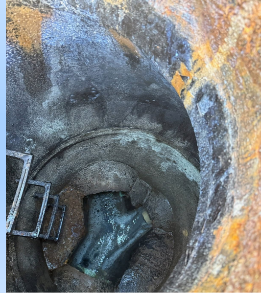
Tie-in of new Seneca Creek force main
