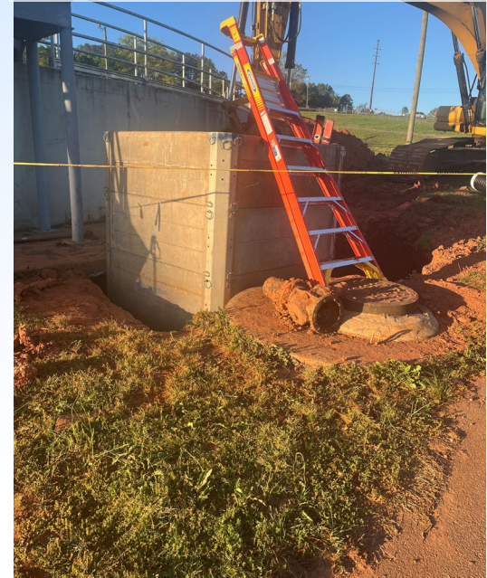
Final Clarifier #3 drain repair
