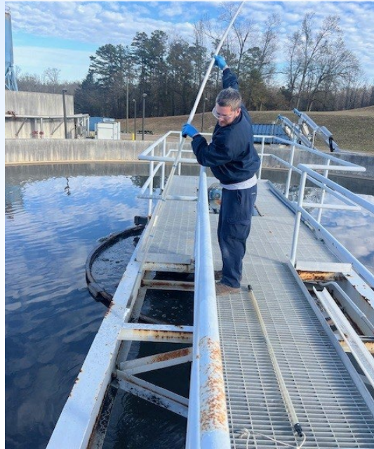
Staff collecting sample from clarifier
