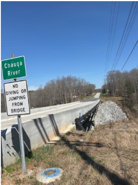
Photopoint 41: 34.68538, -83.15205 View down completed Highway 76 bridge.
