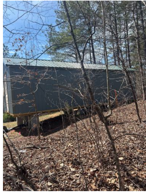
Photopoint 29: 34.69819, -83.15983 New shed likely not on property boundary.
