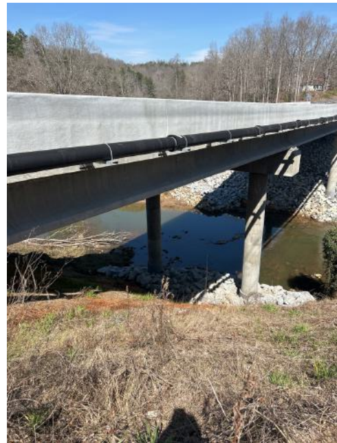
Photopoint 41: 34.68538, -83.15205 View of rock revetments installed below the new bridge..
